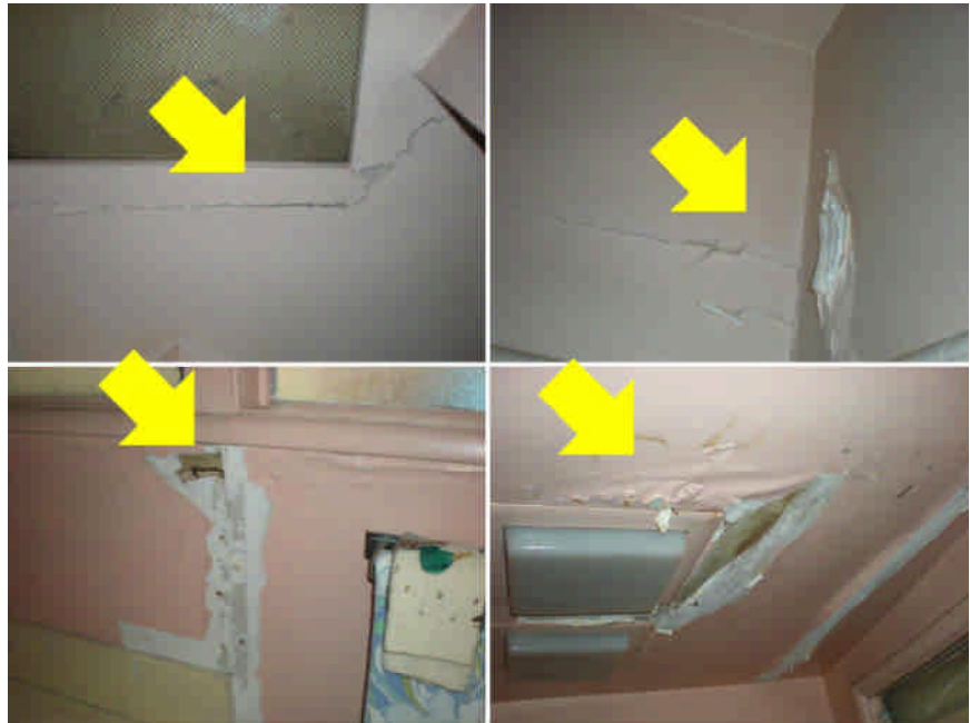
Bathroom # 1: Type: Plaster. Condition: General condition appears serviceable.
