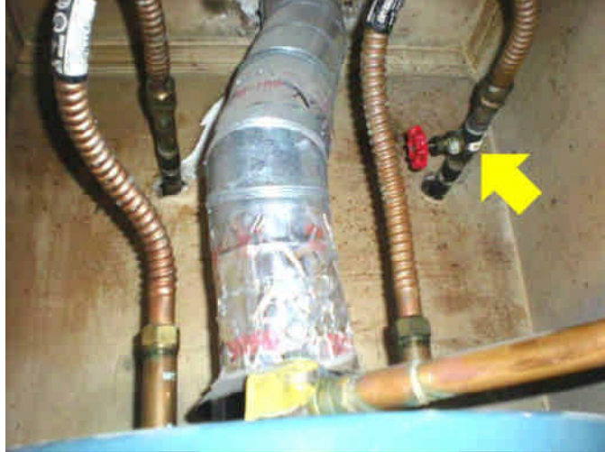
Minor corrosion/rust noted on the water supply lines. See photo.
